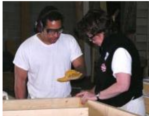
Nancy McLean instructing Louis Thayer on the fine art of building corners.
